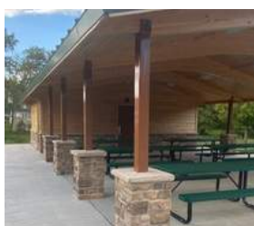
Steel Columns Powder coated steel columns
